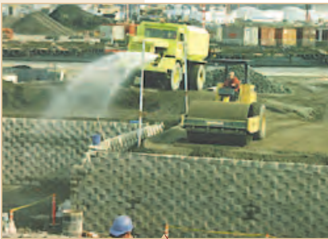
Select Granular Fill With Vibratory Compaction
