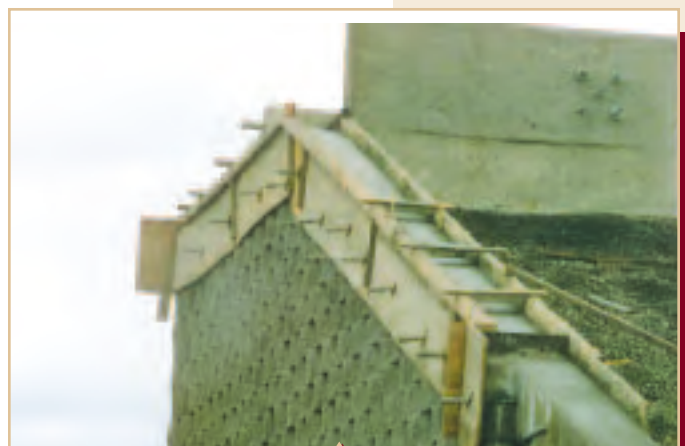
Forming of Site Poured Copings
