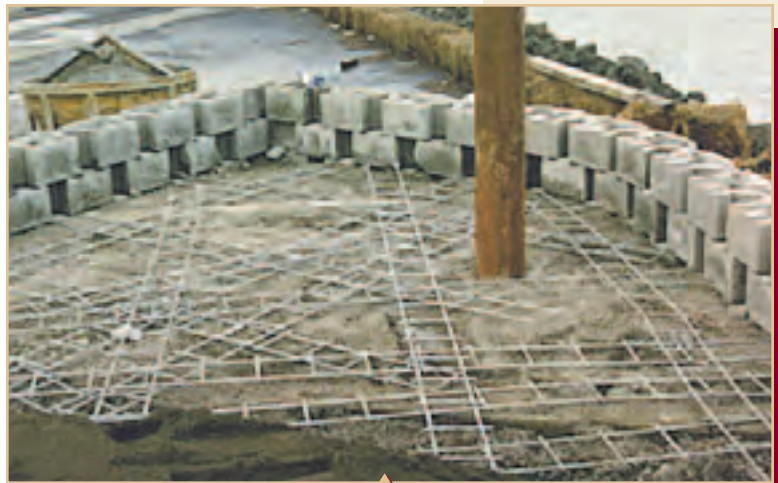
Steel Reinforcing Layout at Bridge Support Point
