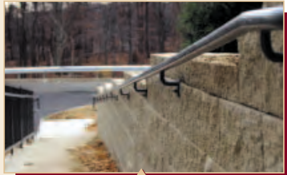
Pedestrian ramp with handrail detailed
