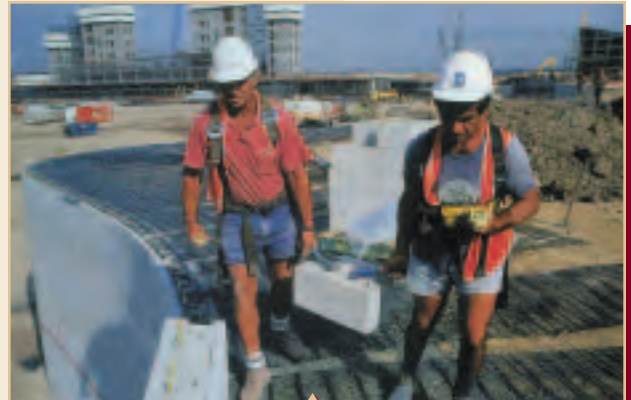
Construction continues with Keystone and geogrid
