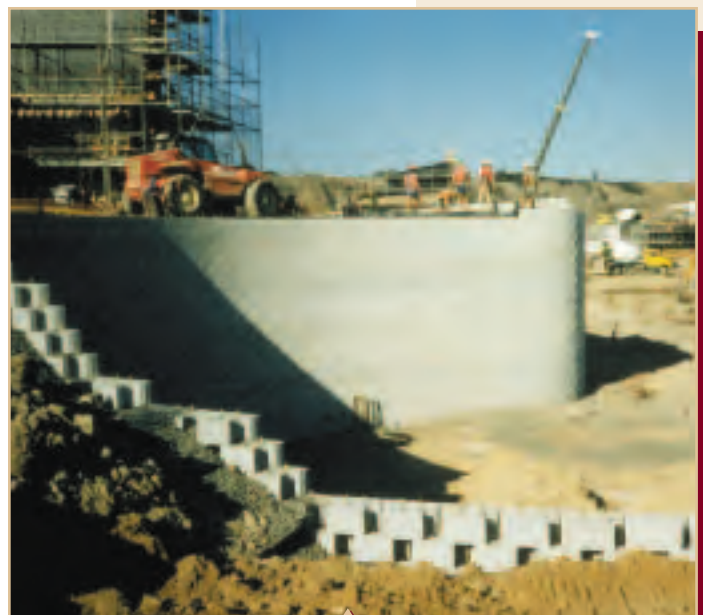
High quality results using smooth texture Keystone units and multiple radii layout.
