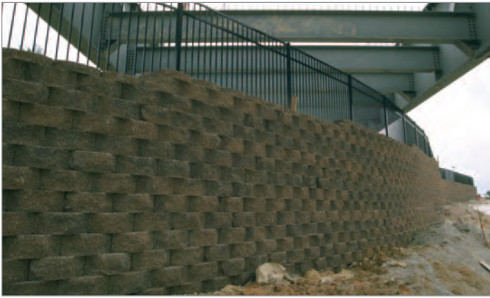
Keystone Compac Tri-plane units were utilized to build this pedestrian walkway.
