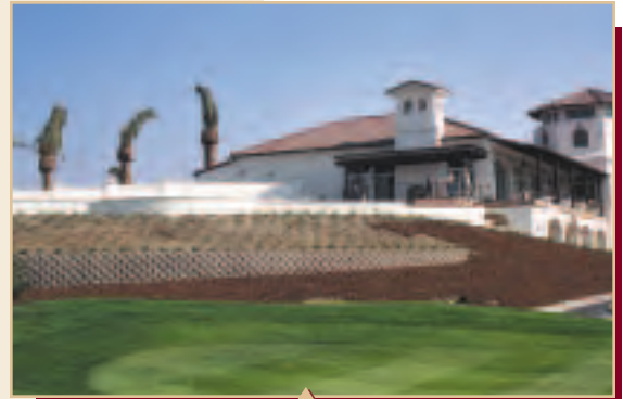
Combination of reinforced slopes and Keystone walls at clubhouse.
