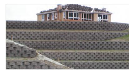
using one strength grid, however some walls are reinforced with up to three different grid strengths. Adapting to the different land conditions required varying grid strengths.
