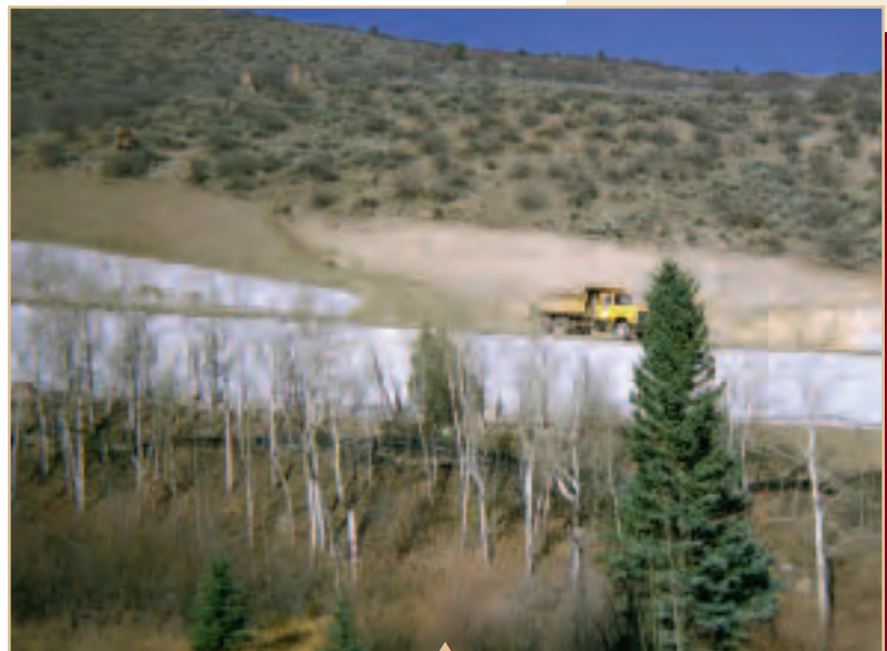
View of completed wall prior to placement of moss stone veneer.
