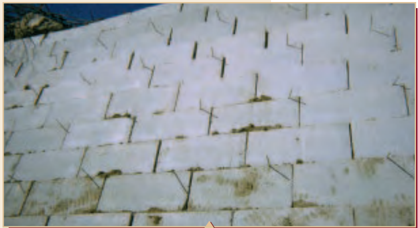
Straight face, unsplit KEYSTONE Standard units with a 9 gauge wire provided the surface and method for attaching the rock veneer.
