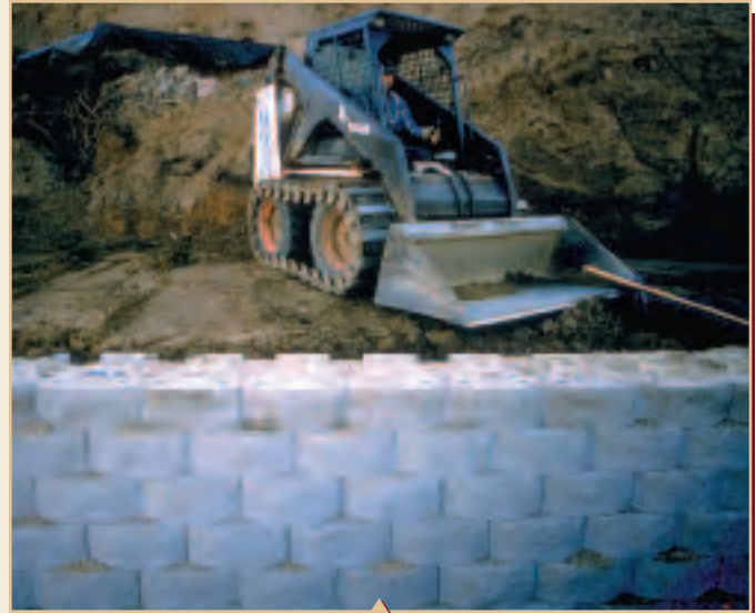
Construction is easily accomplished in tight confines.
