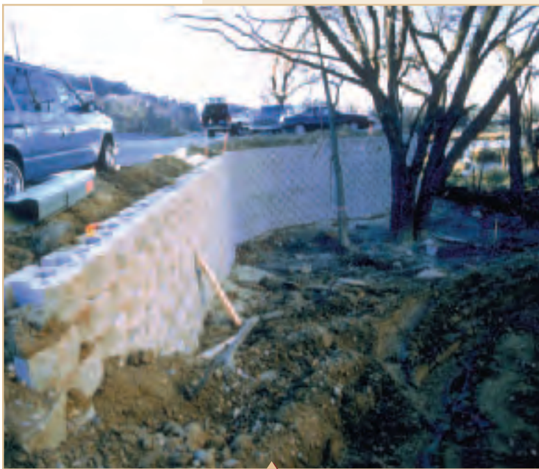
Keystone flexibility allows conformity to site constraints and soft subbase soils.
