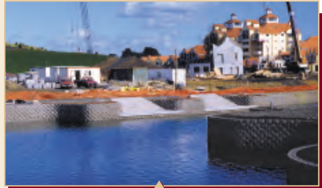
Gulf Harbour site during construction.
