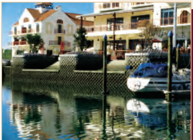
Gulf Harbour Marine Village project with Keystone canal walls.
